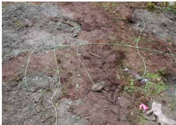
Figure A1.3 Log stringer bridge explosive design. Top: typical explosive placement for removing a log stringer bridge. Middle: Emulsion is well-coupled to sill and stringer logs. Bottom: ANFO is buried in surface decking and primed with emulsion and detonating cord
